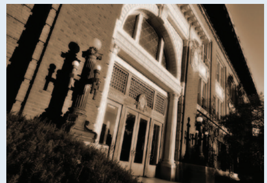
A shot of Lincoln Hall before the renovation work began.
